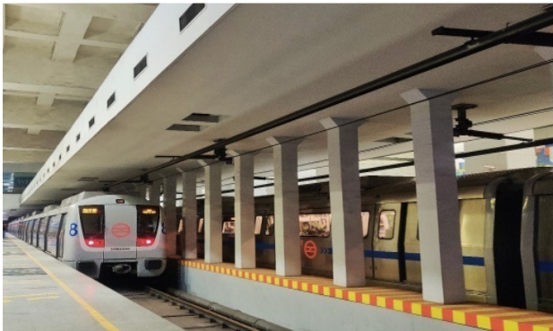
Photo 2: The underground corridor and stations of metro create a parallel city below the traffic snarls and pollution of Delhi roads.
