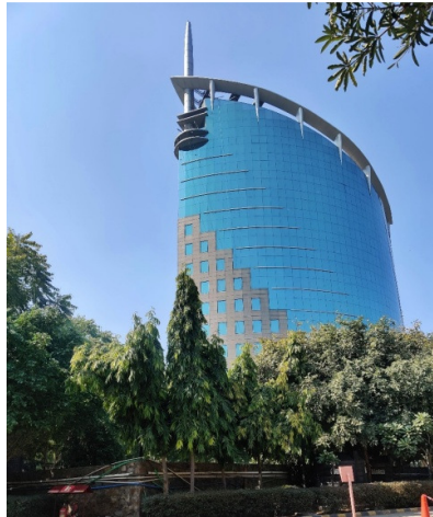
Photo 4: DLF Gateway Tower in Delhi NCR, popularly called the “Titanic”, was designed by Hafeez Contractor. The ship design bears no relevance to the land around.
